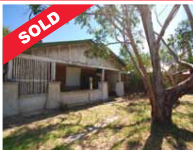
49 Springbank Road, Colonel Light Gardens
